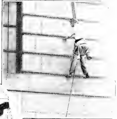
Adjustable stirrups hang from the front of the chair and enable the painter to stand up when he wishes
